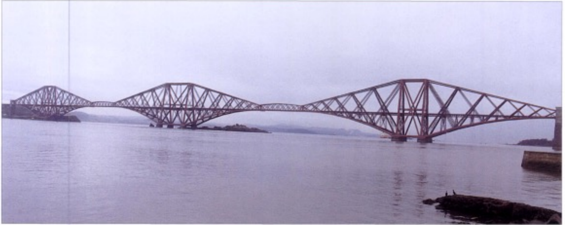
Figure 6.12 Forth bridge in Scotland, two main spans of 521 metres (1890), J. Fowler and B. Baker.
