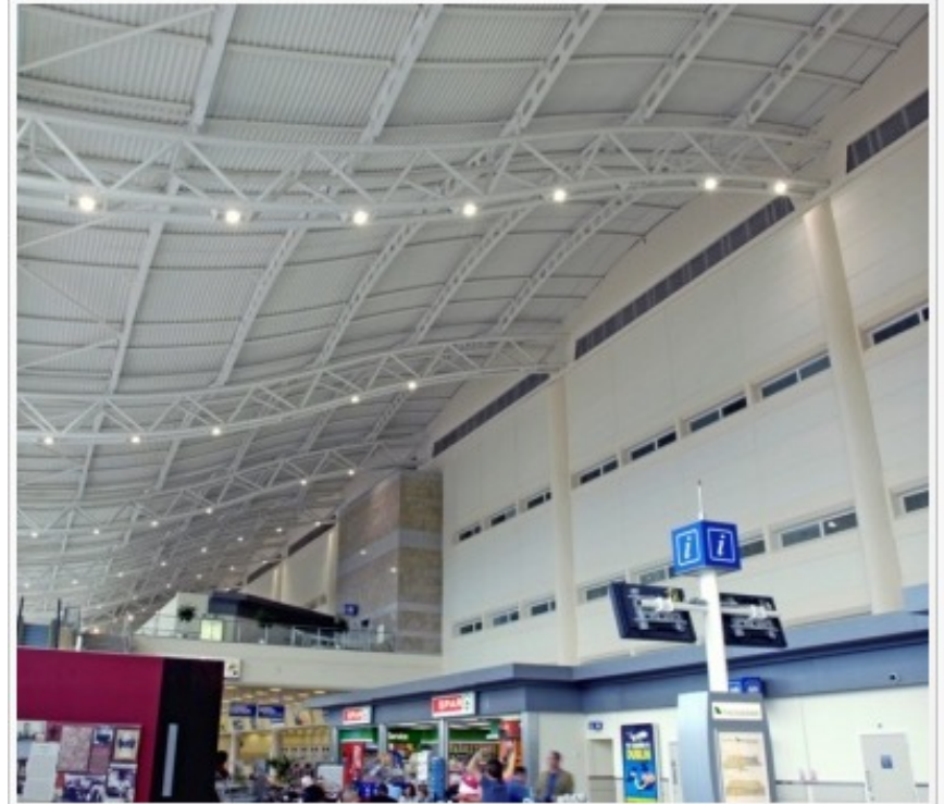
Long-span, curved roof trusses Robin Hood Airport, Doncaster
