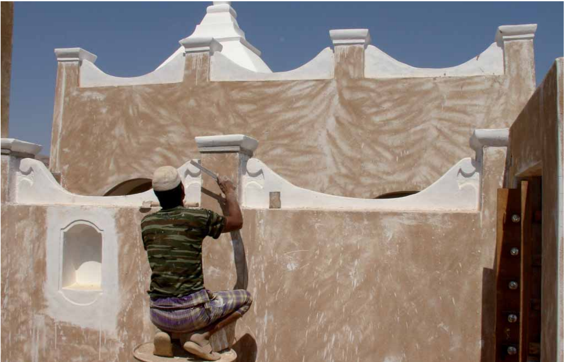
Ba Ziad mosque, during restoration.
