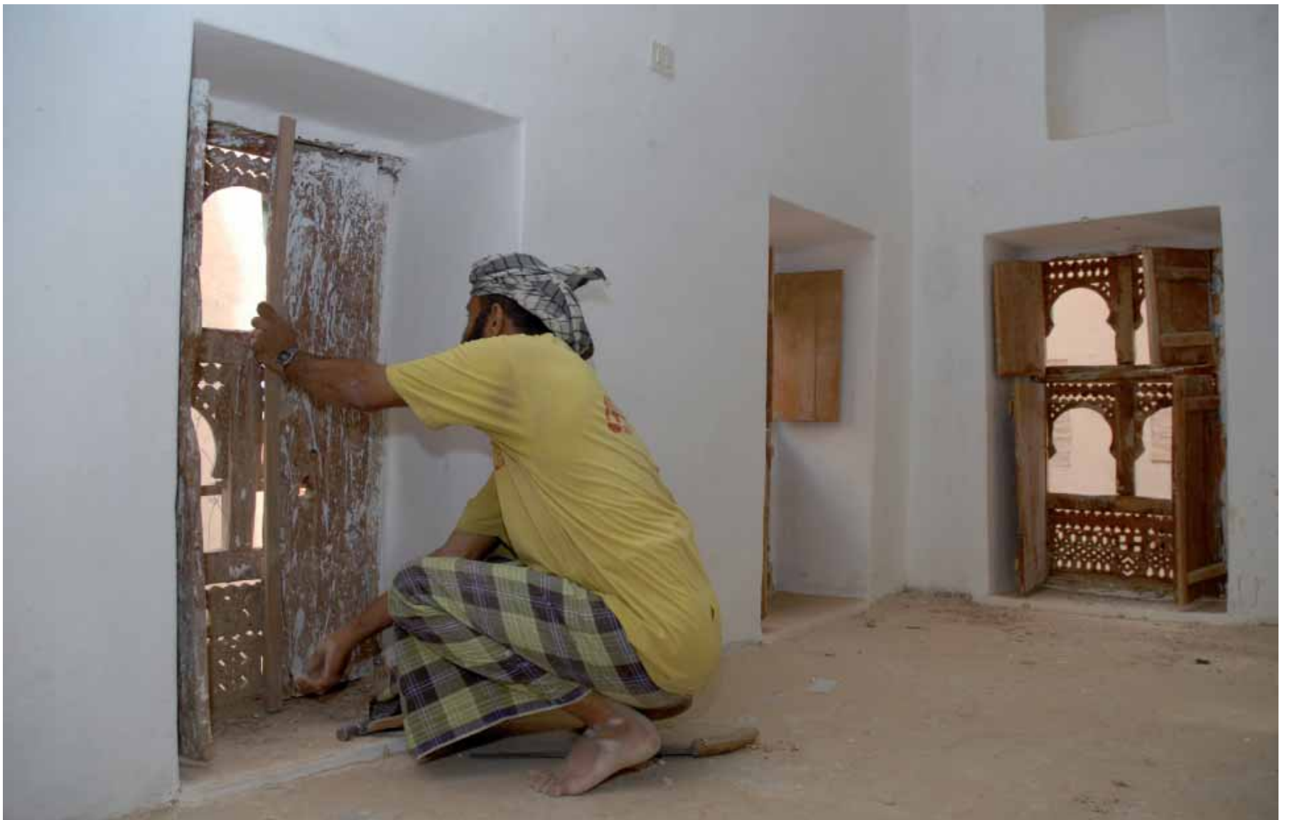
House D56, restoration of wooden window.
