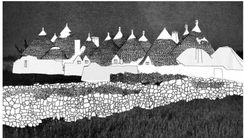
Fig. 18-20. Trulli at "water out", the drainage lines of the roof and the ground carry the water to a well or to an outdoor cistern to the house. This water serves the neighborhood (author: G. Mazzone)
