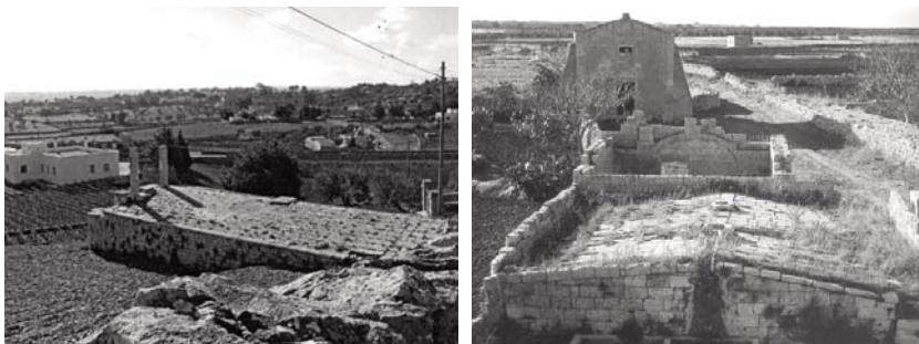
Fig. 6-8. Model and images of rural semi - hypogeal cisterns with trough typical of the "murgian" country. (author: C. Montalbano)
