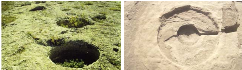
Fig. 4-5. Micro-cisterns: water structures diffused on the Apulian limestones plateau and their similarity with those present in almost all the Mediterranean area (in photo 6: Petra) (source : P. Laureano, I Giardini di Pietra. I Sassi di Matera e la civiltà Mediterranea , Bollati Boringhieri, Torino 1998)
