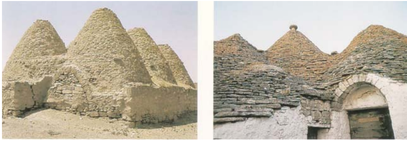
Fig. 24-25. Morphological analogies in the Mediterranean ambit among structure to pseudocupola: the habitation of Harran (Turkey) and the "Trulli" of Alberobello (source: P. Laureano, "Giardini di Pietra")
