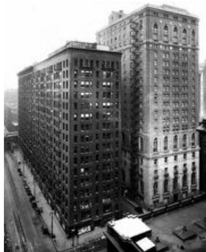
Burnham & Root – Monadnock Building, Chicago 1889-93
