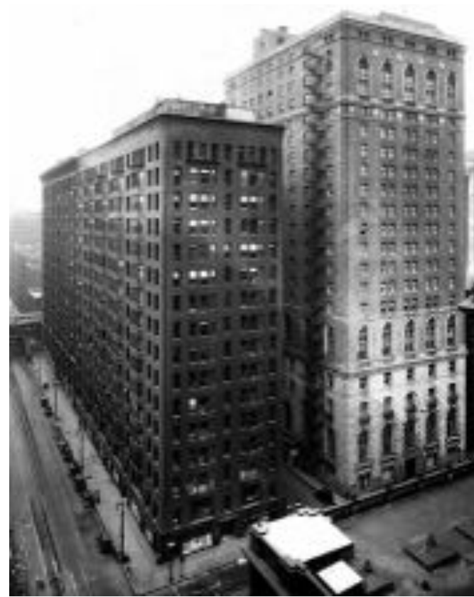
Burnham & Root – Monadnock Building, Chicago 1889-93
